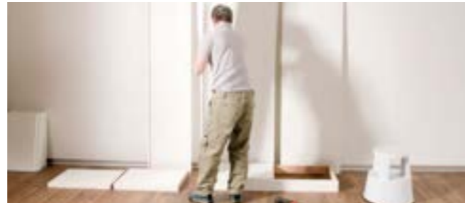
Place furniture side on base. The element is correctly positioned by the protruding screw.
