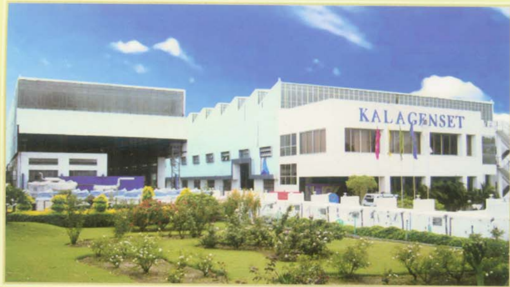
KALA GENSET PVT. LTD. Factory, Chakan
